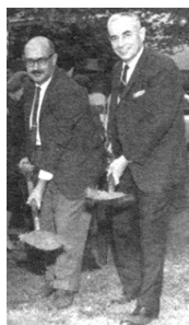
Jaffe and Orchin initiating construction of Crosley Tower
